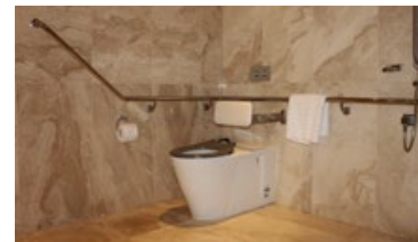
The toilet has grab rails and a backrest.
