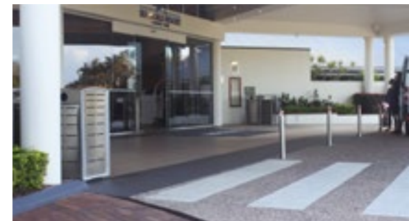
The drop off point has flat, covered access.
