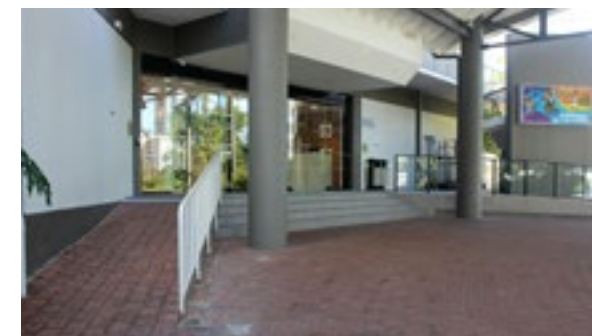
There are ramps to the main entry.
