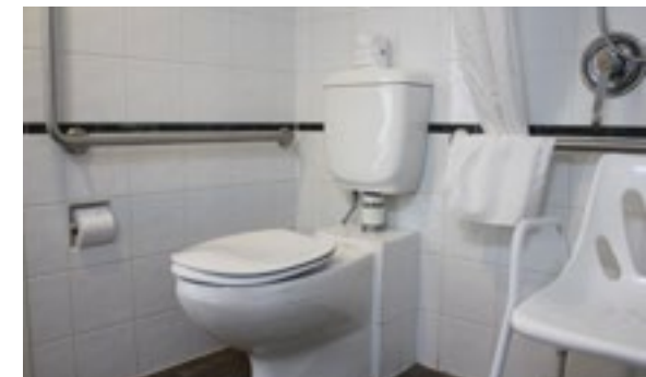
The toilet has grab rails.
