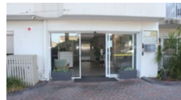
The entry has automatic doors.
