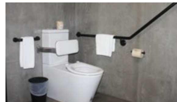
Accessible toilet in the QT cabins
