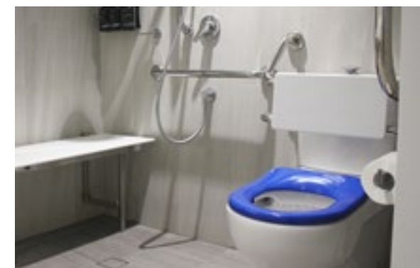
The toilet has grab rails and a backrest.
