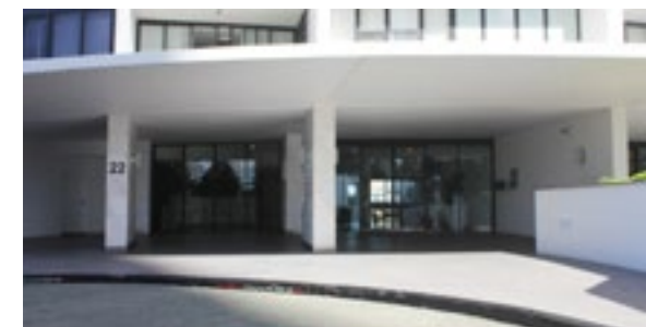
The entry area has double, automatic sliding doors.
