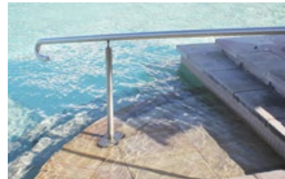
Handrails lead into the outdoor pool.
