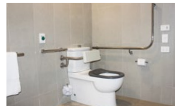
The toilet has grab rails and a backrest.
