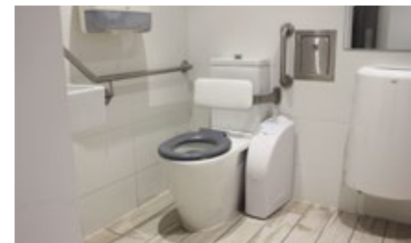
The common area toilet has a side handrail and backrest.
