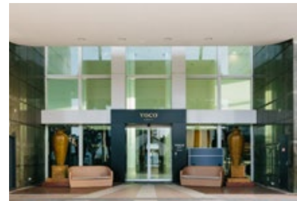
Automatic sensor doors at the property entry.
