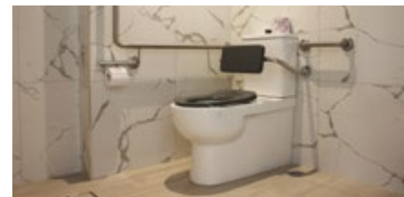
The toilet has grab rails and a contrasting backrest and toilet seat.
